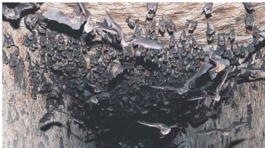
A colony of Hipposideros ruber bats hanging from the roof of a road culvert on São Tomé near Praia Mutamba. Years of bat residency have left a springy, stinky layer of guano underfoot.
