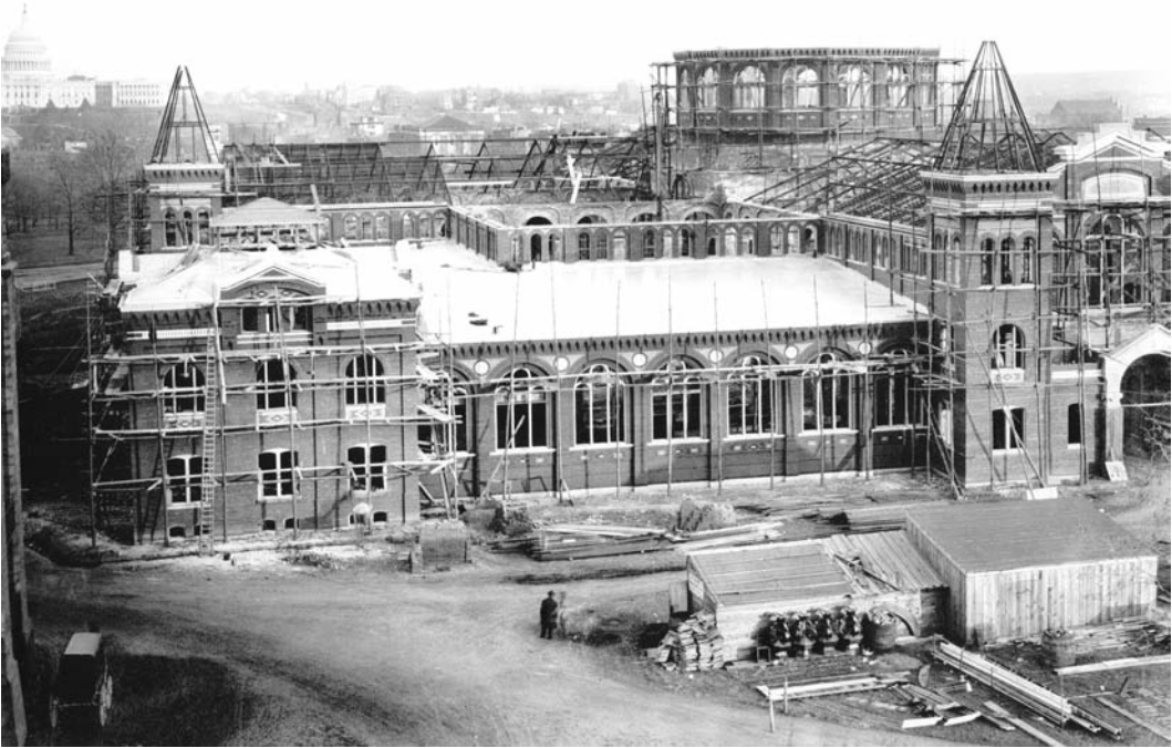
FIGURE 8. The United States National Museum under construction; the entrance, flanked on either side by a modest spire, is partially shown at the right. (SIA Negative number 2003-36480.)
