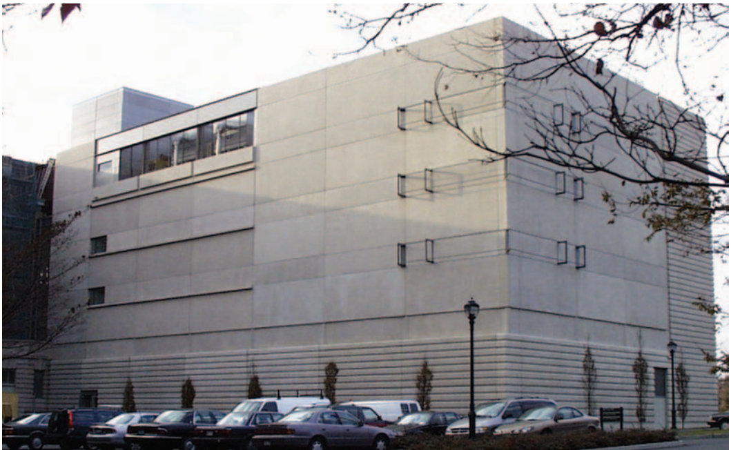
FIGURE 1. Exterior view of the new wing for botanical collections at the New York Botanical Garden, New York City. Photo by author.
