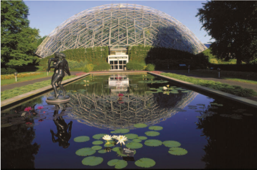
FIGURE 2. The Climatron, completed in 1960, displays tropical plants. It was the first use of a geodesic dome as a greenhouse.
