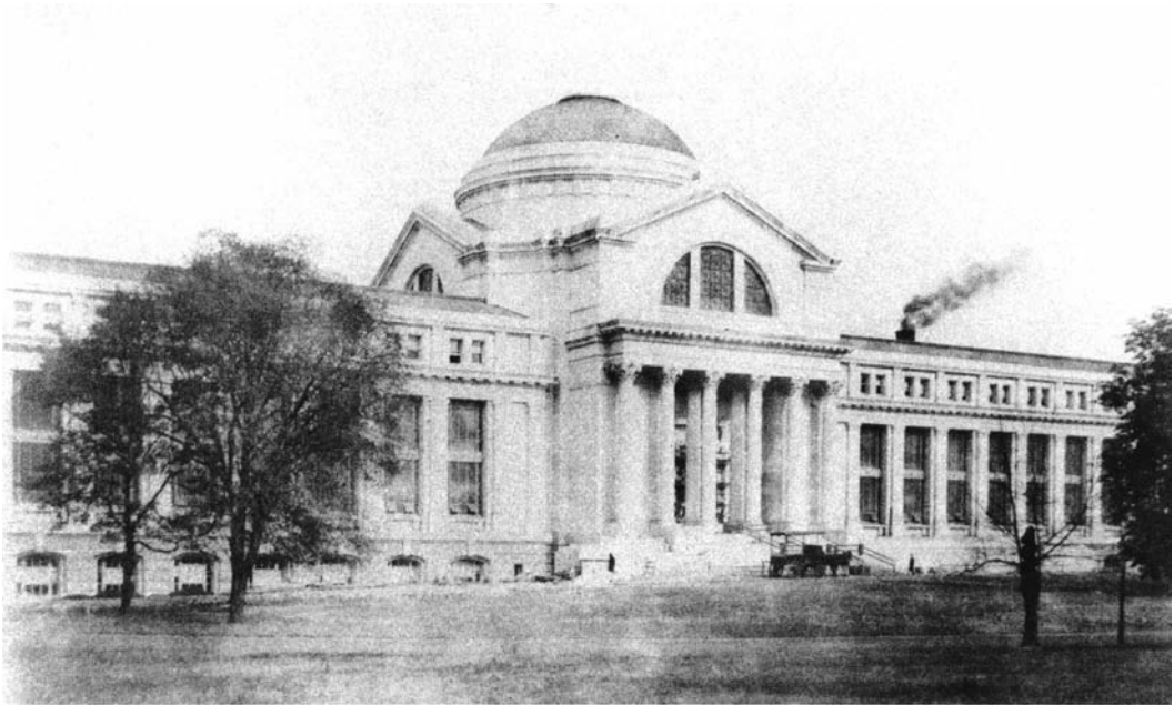
FIGURE 16. The new natural history building in 1909, looking northeast, with a wagon in front and with work continuing on the roof. For several generations this was almost always referred to as the New National Museum. (SIA Negative number 87-4899-20.)
