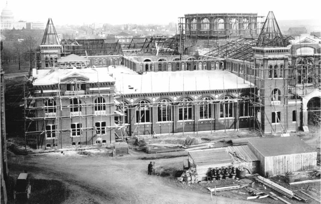
FIGURE 8. The United States National Museum under construction; the entrance, flanked on either side by a modest spire, is partially shown at the right. (SIA Negative number 2003-36480.)
