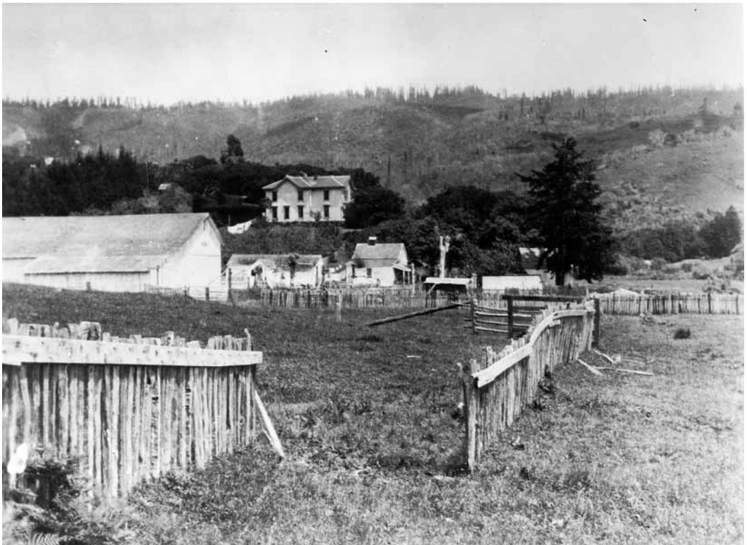
FIGURE 13. Fence offset 8.5 feet. Trace of fault barely visible, running from lower right to upper left through offset. Photograph by G.K. Gilbert. (G.K. Gilbert Collection [N7583-C], California Academy of Sciences Archives.) (Also in Gilbert 1907b, pl. 1, fig. B.)
