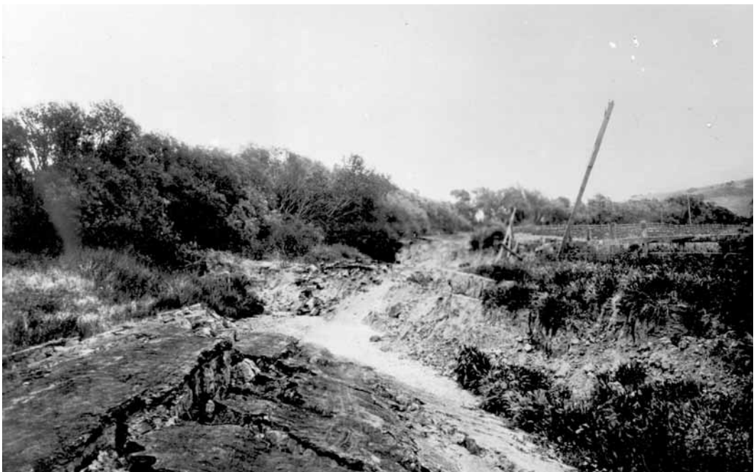
FIGURE 12. Road bed between Olema and Inverness. Road bed probably destroyed by shaking of soft ground beneath. Photograph by G.K. Gilbert. (G.K. Gilbert Collection [N-7583-F], California Academy of Sciences Archives.)
