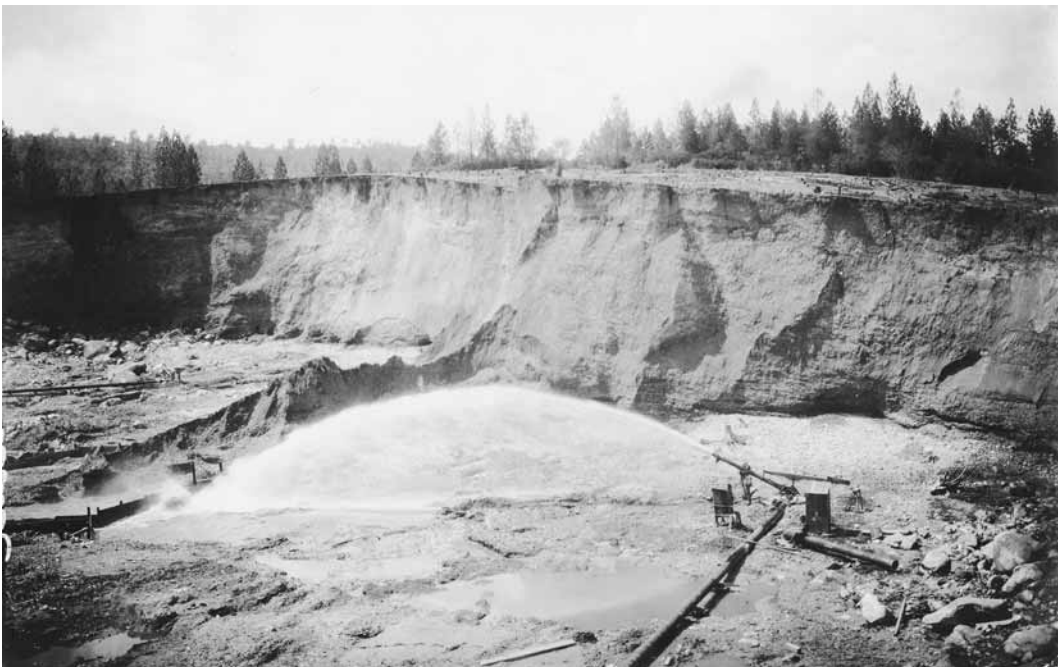
FIGURE 4. Hydraulic mining at the Esperance Mine, French Corral. Photograph by G.K. Gilbert. (G.K. Gilbert Collection [331.1.6.1; envelope #4], Alice Eastwood Archive, California Academy of Sciences Archives.)
