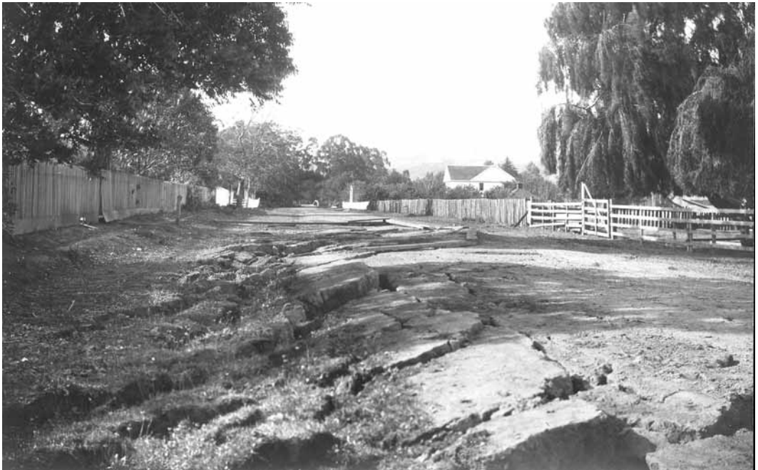
FIGURE 21. Branch of fault-trace in north part of Bolinas, looking NNW, illustrating diagonal cracks. Photograph by G.K. Gilbert. (G.K. Gilbert Collection [331.6.1, #165; Unnumbered white envelope], Alice Eastwood Archive, California Academy of Sciences Archives.) (Also in Gilbert in Lawson 1908, pl. 39, fig. A).
